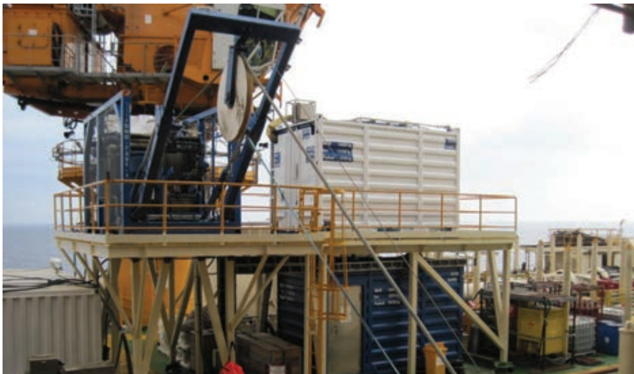
The containers hold equipment and controls used for dual-gradient drilling off of Cuba by Petronas. Courtesy of Petronas.
